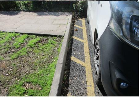
The side of the bay showing insufficient space for a passenger to transfer and no dropped kerb access
