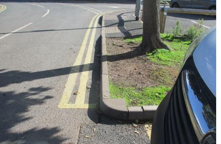
The ground alongside the bays showing no dropped kerb access and an uneven, muddy verge
